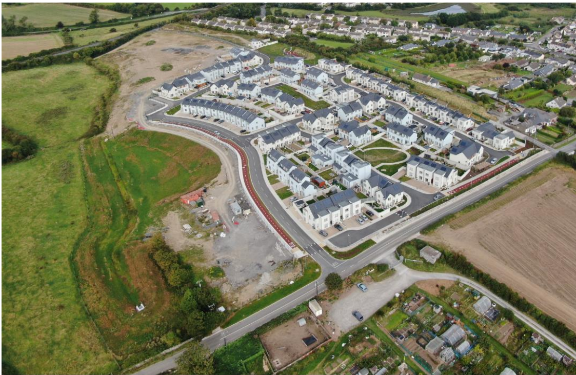
Figure 3: Partially Constructed RDF
